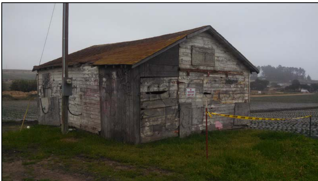
Figure 2-1: Existing Springfield Well Site
